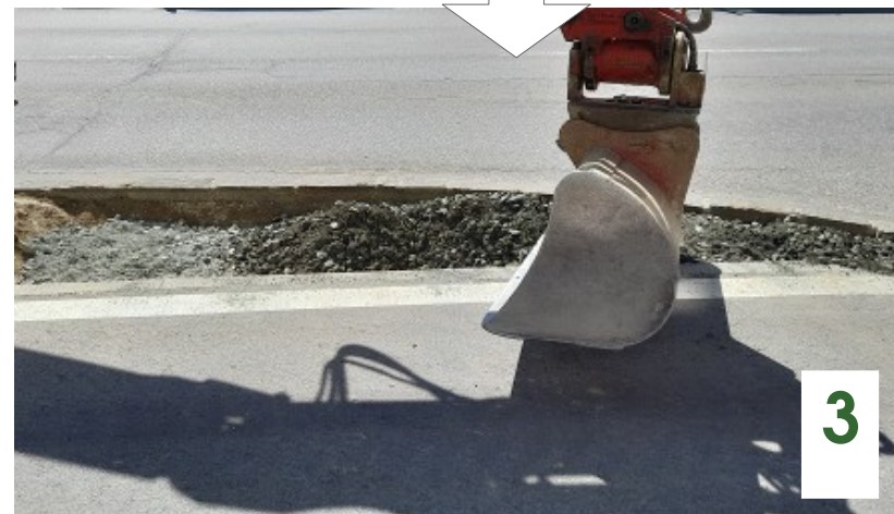
Adding the second layer of gravel and compost
