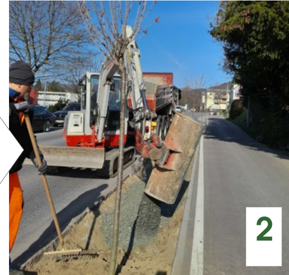
Adding the first layer of 0-30 coarse gravel
